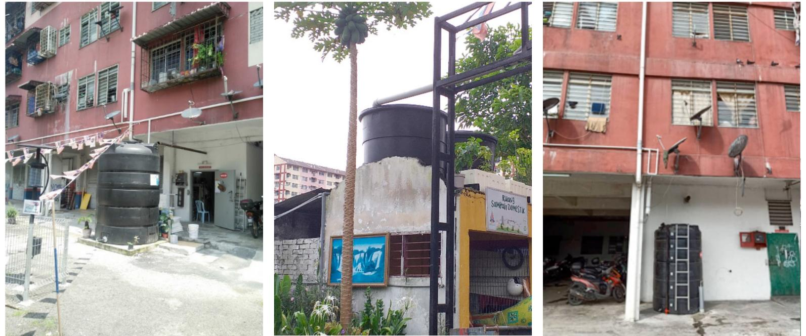
Figure 4. Rainwater harvesting systems in Sungai Penchala basin
